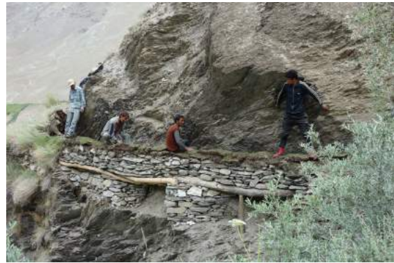
Photo 2: Villagers repairing an irrigation channel in Ladakh, 2013
